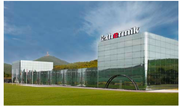
Thermik headquarters, Thuringia (Germany)
